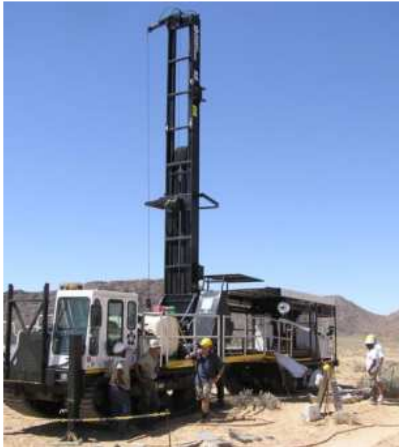
Figure 10-3. Boart Longyear Sonic rig drilling at Henkries Central.
